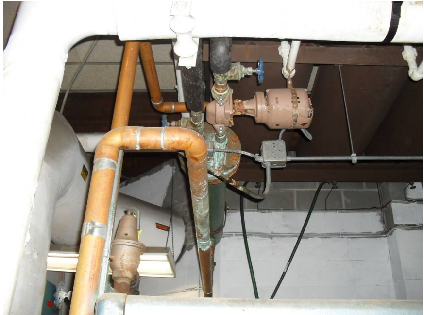
Figure 9 - DHW shell &amp; tube heat exchanger
