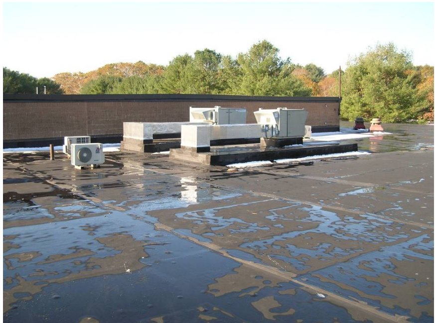
Figure 7 – Typical new Energy Recovery ventilators
