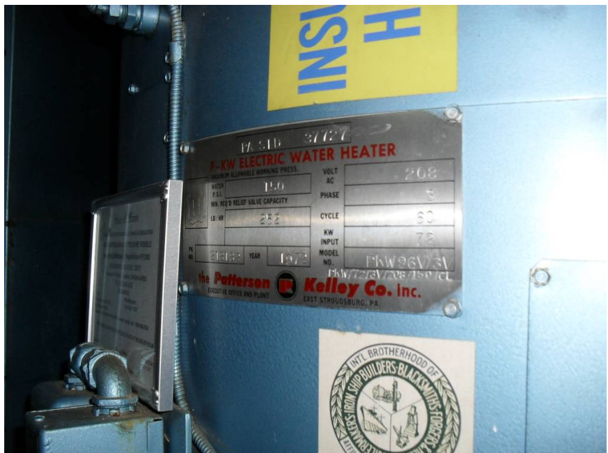
Figure 10 - 72 kw electric water heater
