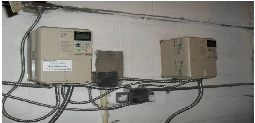
Figure 5 – Base mounted pump variable speed drives
