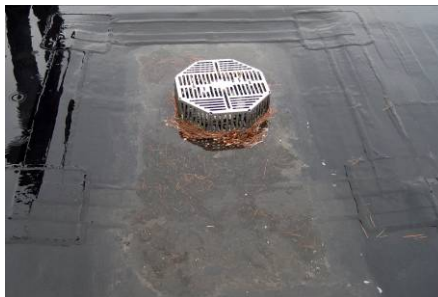
Typical roof drains set in sumps
