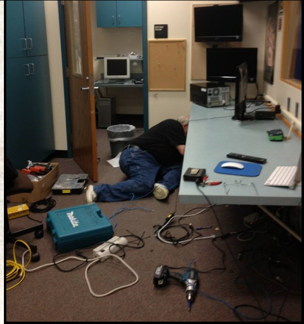
Robert, the installer and trainer, was here from 8a.m. to 5 p.m.
