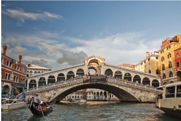
The Rialto Bridge and the Grand Canal, Venice
