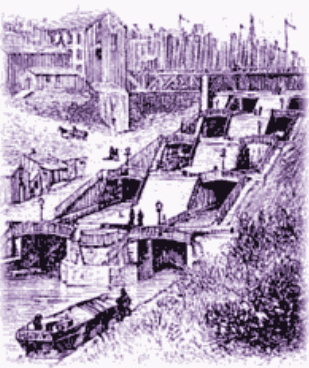
Locks like this one on the Erie Canal made it possible to connect the Hudson River and Lake Erie despite their 571-foot difference in height.
