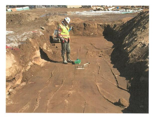
Density testing of granular borrow at section AC foundation.
